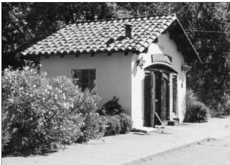
Figure 3-5 View of warming house from north.
